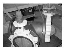
Step 6) There are no other possible orientations of this bracket. The Master crank arm will rotate 90 degrees clockwise, and there are reliefs in the sides of the bracket to accommodate this angular rotation.
