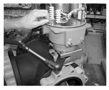
Step 25) Using the correct control signal (On/Off or Proportional) drive the MASTER valve 25% CLOSED, then drive the MASTER valve fully OPEN. The SLAVE valve should now be fully CLOSED. The SLAVE valve should now be fully CLOSED. If the
